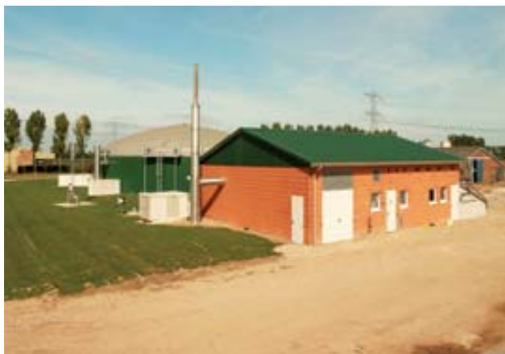
The technical building and the fermenter. It has a net volume of 3,4000 cubic meters.
