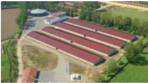
The biogas plant in Casaleto Ceredano.
